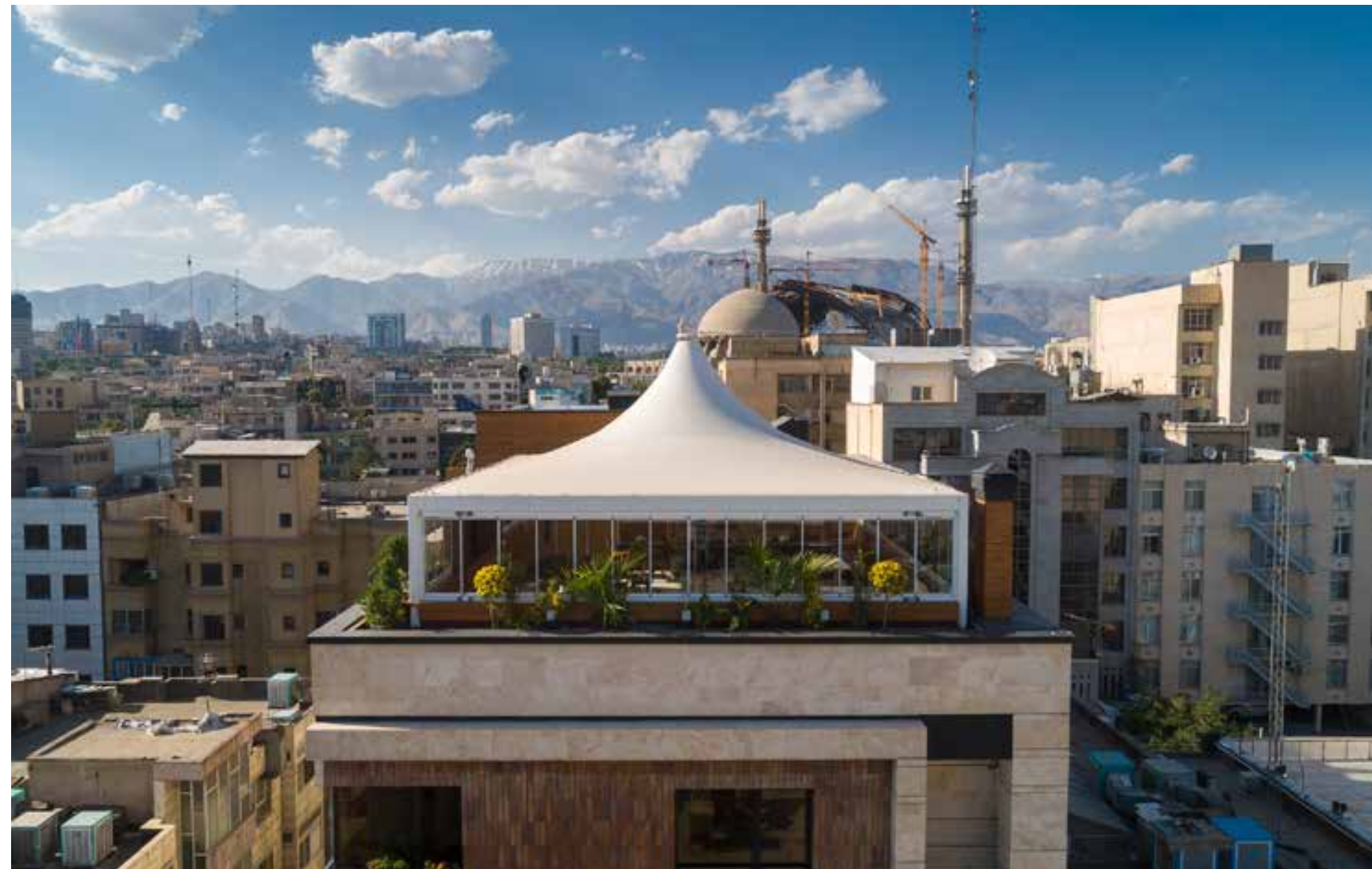
Membrane Canopies Motahari Roof Garden Tehran
